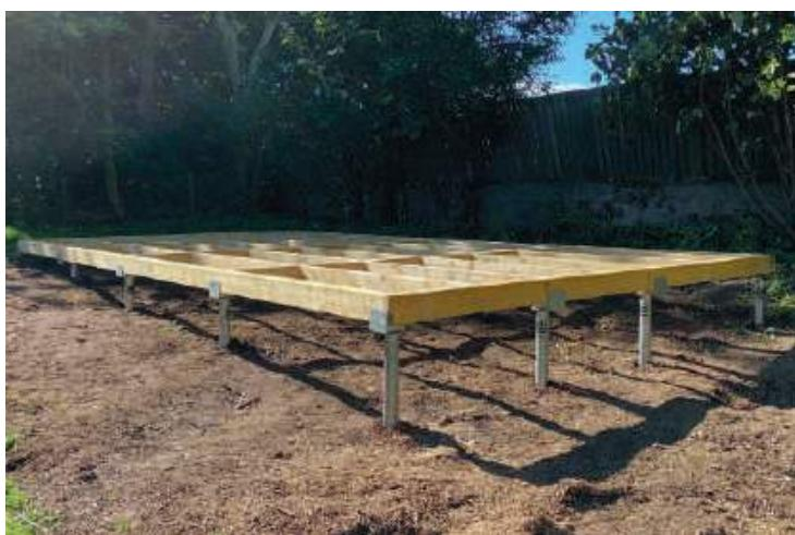
**EN** metal screws option - higher cost solution but no need for earthworks
